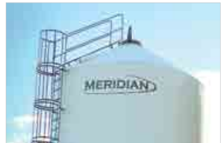
LADDER CAGE & HANDRAILS
