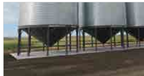
CUSTOM CONCRETE FOUNDATIONS
