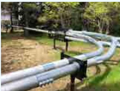
All the working components on the ground!
